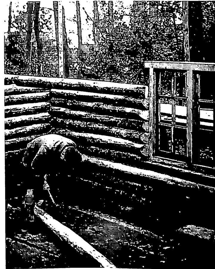
BUILDING THE LOG CABIN AT GILWELL PARK
