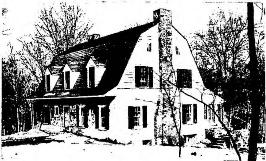
A modern home near Washington, D. C. to the eye, yes. But its first story walls are made of rammed earth. Below are the rammers made by a present day blacksmith which were used in tamping the walls of this modern pisé home.
