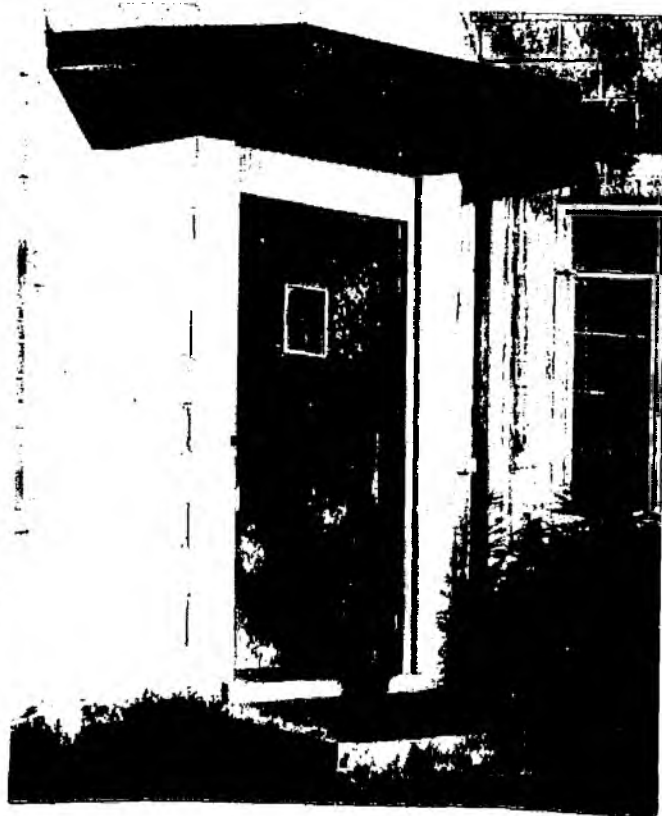
Modern as tomorrow is this straight, simple doorway in the modern house. It makes no pretense at being anything but a utilitarian door, it is sheltered because that is more practical and it introduces no new material in its decorative scheme. The glass is advantageously placed to give the occupant of the house a view of the steps and all callers.
