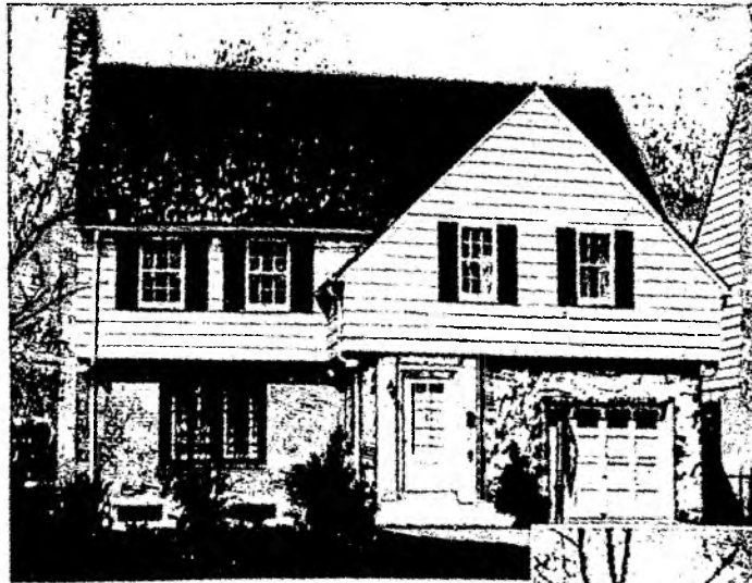
Left—Combinations of three structural and decorative materials—siding, stone and brick—make the face of this house different and interesting. Because it serves a modern family, the garage is a part of the house.
