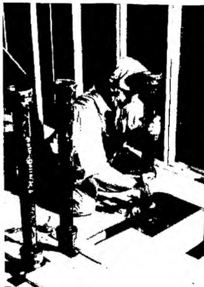
Major repairs are necessary only occasionally in the life of the well built home, but they must be considered.
