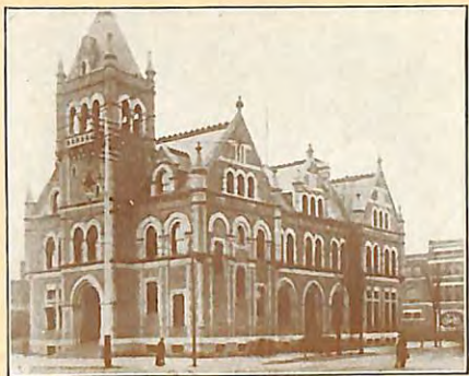
Old Post Office at Fifth and Main. Now Fidelity Building.
