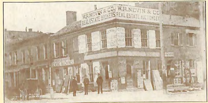
North East Corner Third and Jefferson Streets 1880. Now Beckel Building.
