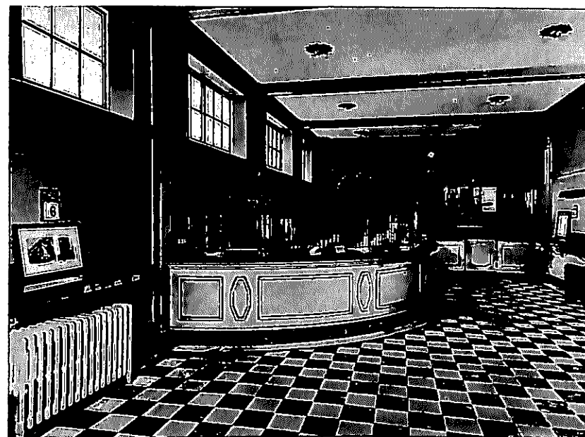
INTERIOR OF ROSLINDALE BRANCH 754 South Street, Roslindale.
