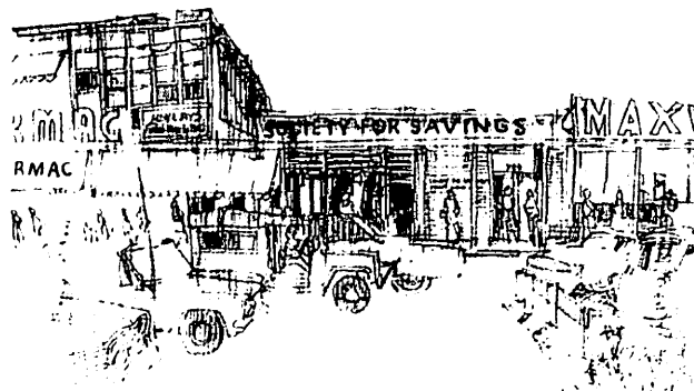
Bishops Corner Branch Office, 1957
