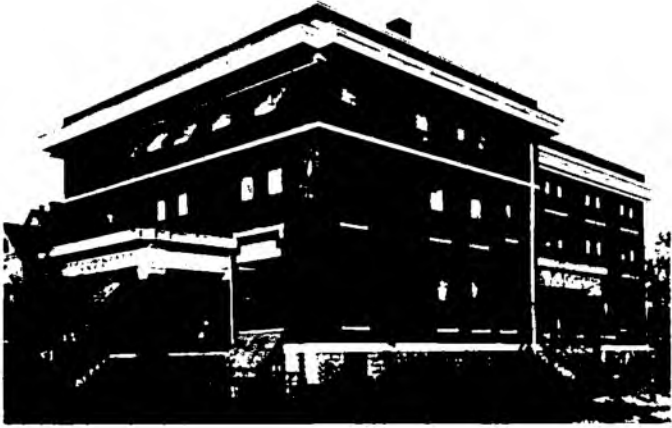
RAILROAD "Y" BUILDING AT LOUISVILLE, KY.
