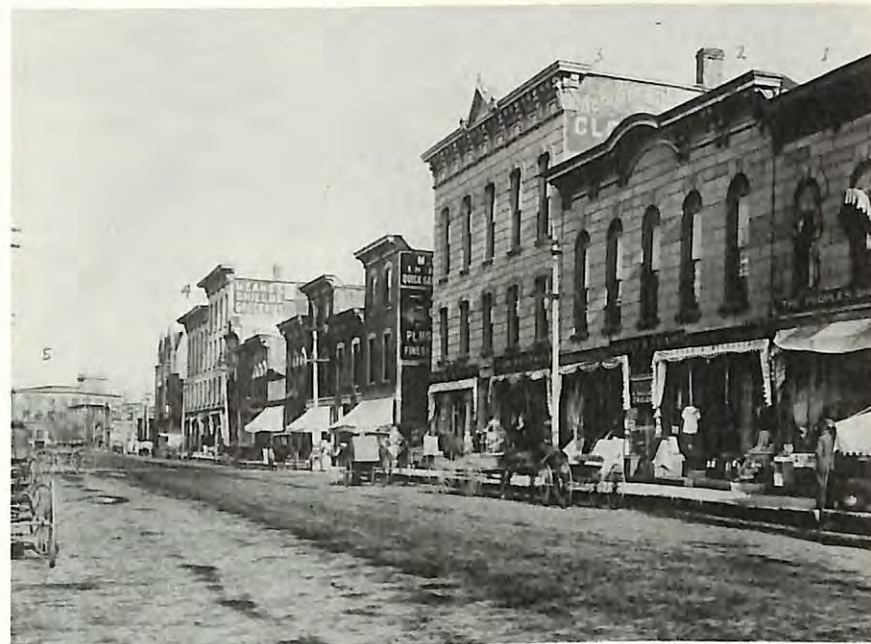
River Street in 1886. Our River Street building was #2. Hopkins law office was in #3. Old Dunning block #4, and Cotton Mill building #5. Some say Hopkins had an office in #1 at one time.
